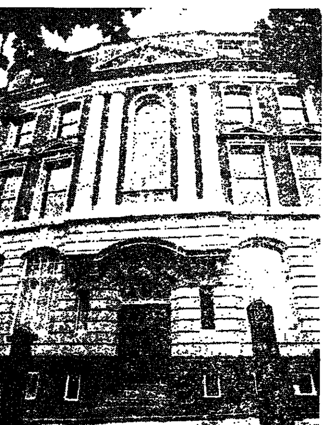
Haslemere Estates has just completed the refurbishment of West India House and 54 Baldwin Street, Bristol. It comprises 11 offices suites, ranging from 800 sq ft. The building which is on the Quay side, is close to Bristol's financial centre. Hartnell Taylor Cook.
